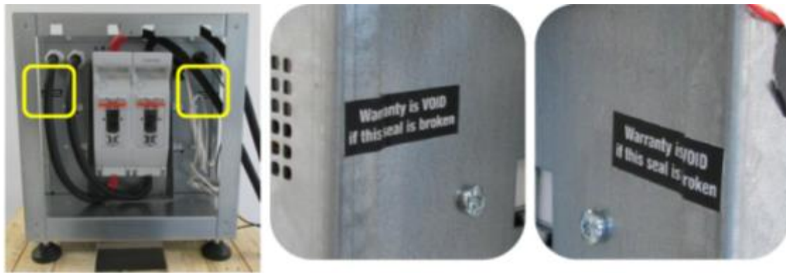
Figure 3-2: seal position
